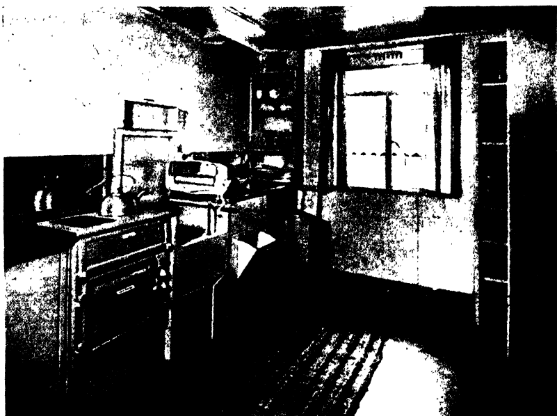
Prefabricated Kitchen Unit in the Aluminium House, Showing Refrigerator, Cooker, Wash-Unit, Cupboards, etc. (With acknowledgments to the Ministry of Works.)
